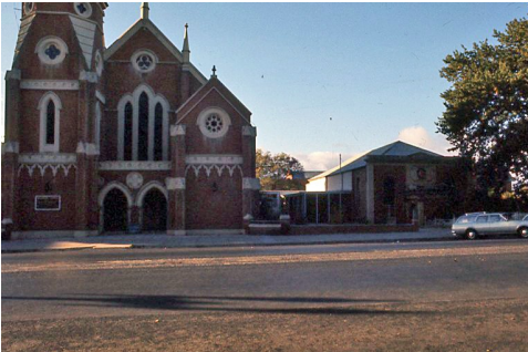
Methodist Church, Bathurst, NSW
