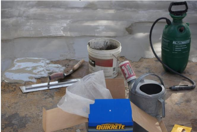
I mixed the concrete powder (from blue box) with water in small batches and poured it on the floor. Then I smoothed it with the flat blade. I had a tank (green) of water for spraying the floor to make a wet contact. The watering can had water to add to the concrete powder. I mixed them in the white bucket.
