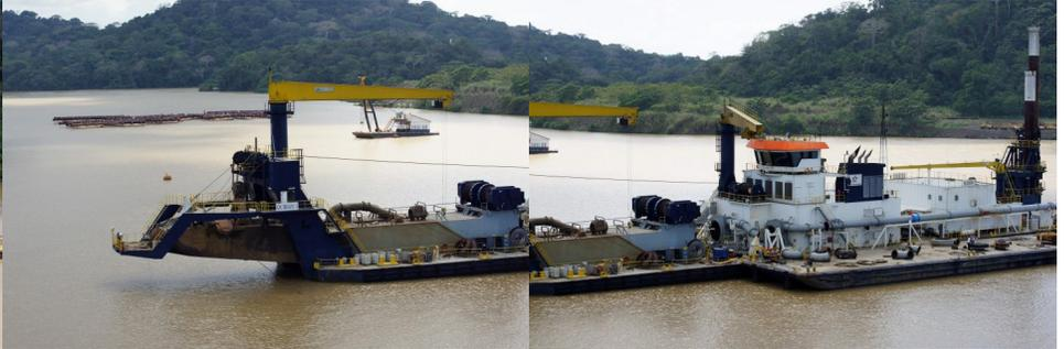
The canal is being dredged to make room for larger ships. Some equipment loads debris onto barges, as at the left. Other equipment continuously digs sediments and pumps them to the shore using large pipes, such as those rafted in the background of the middle photo. Several times we saw trains on the east side of the canal carrying containers between the port cities. The white tower behind has ship navigation aids.
