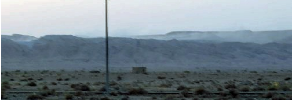
Blowing dust from the Gafsa phosphate mine.
