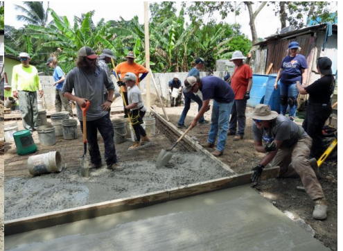
Concrete floor smoothing progress
