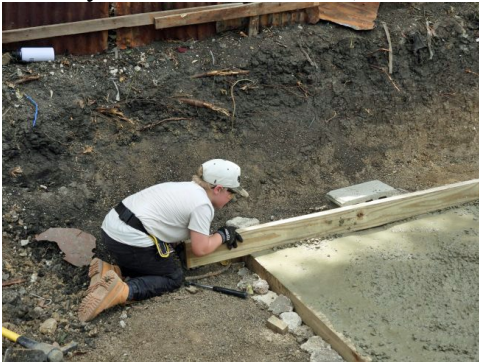
The leveling board is sawed back, forth
