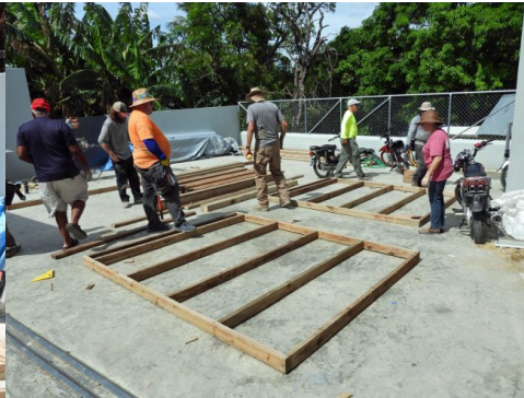
Building the walls
