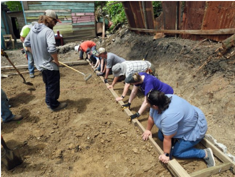
Determining the level of the clay floor
