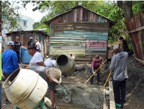
Initial concrete dump raked to edges
