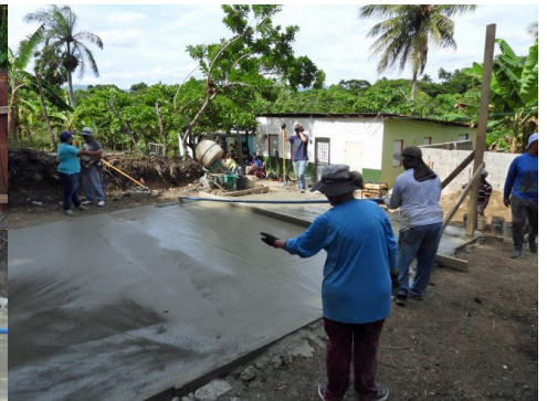
Almost done pouring concrete
