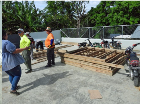
Stacking the walls
