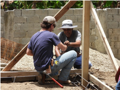
The corner post holds up the patio roof
