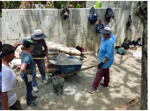
Loading buckets with cement
