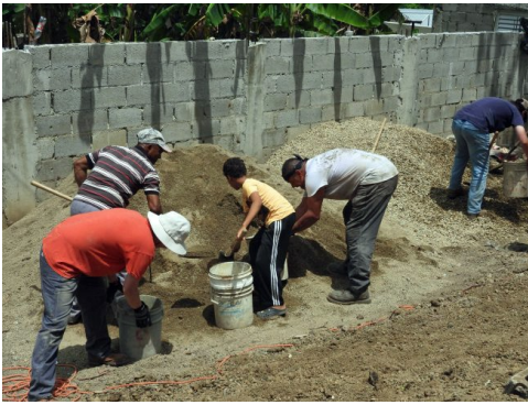
Loading buckets with sand
