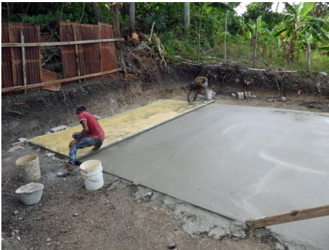
The concrete finishers add yellow dye
