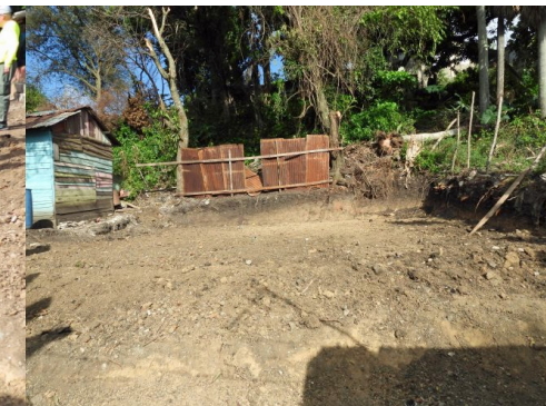
View west: leveled home site
