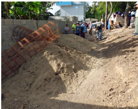
View south: sand, gravel, rebar
