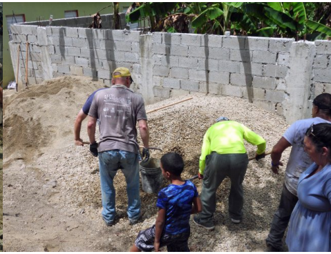
Loading buckets with gravel
