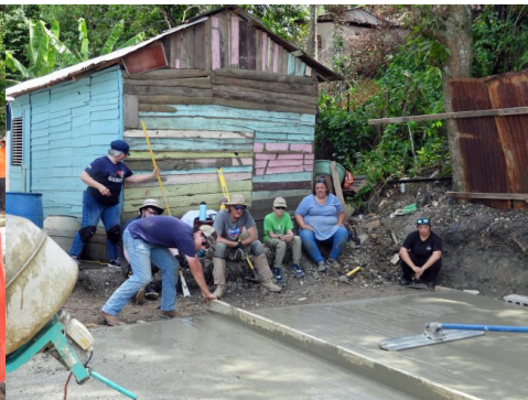
Leveling and smoothing the concrete
