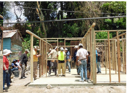
Inserting front entrance wall
