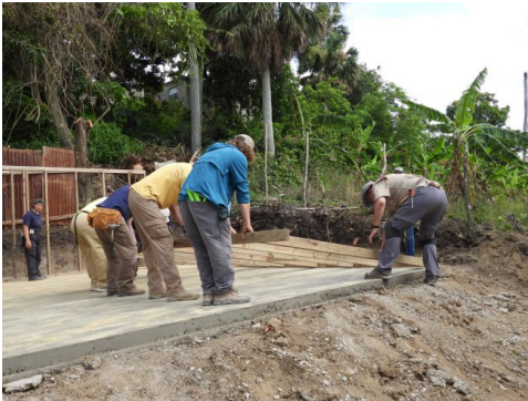
Laying it down for splicing
