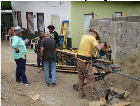
Cutting siding boards
