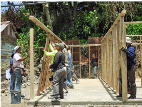
Raising south wall
