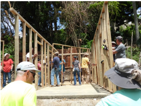
First bedroom wall inserted
