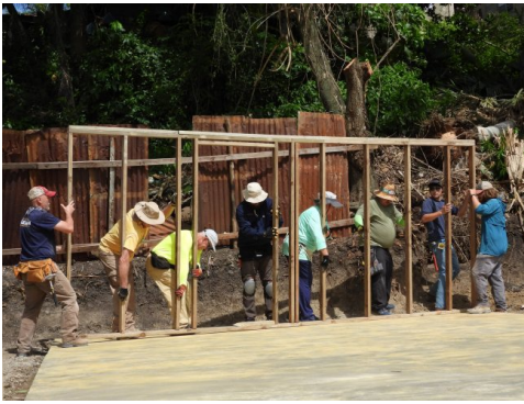
Back wall positioned
