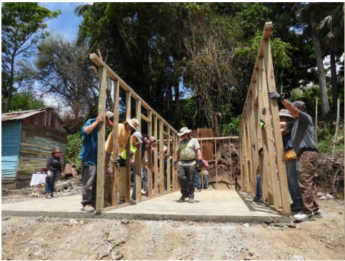
Positioning the middle wall
