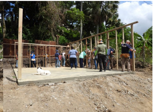
Positioning and joining north wall
