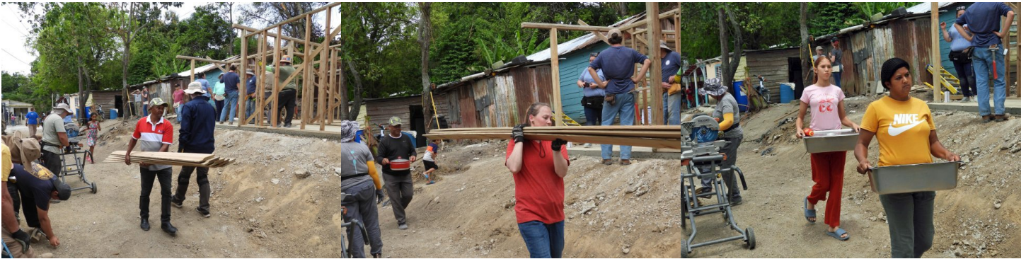
Siding boards were brought next
