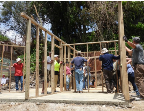
Second bedroom wall inserted
