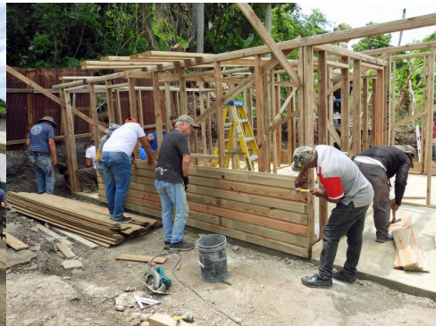
Rafters stacked on top
