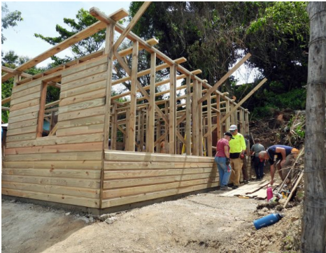
Rafters loose in place, not yet vertical
