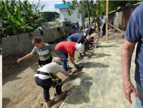
Removing front form
