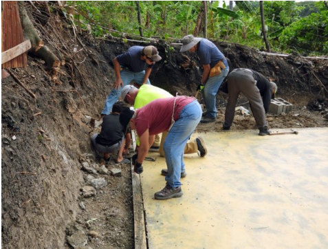
Removing back form
