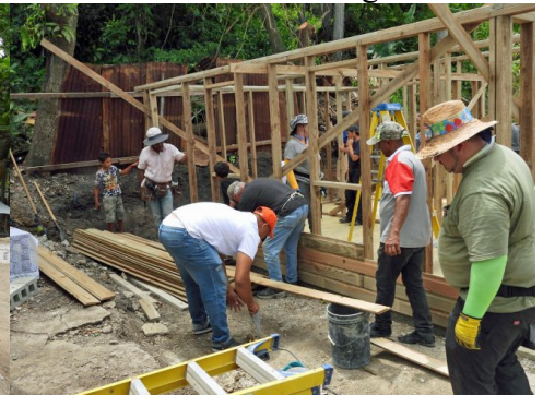
Measuring for circular saw cut of siding
