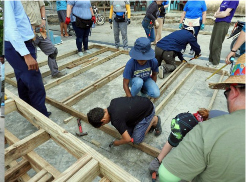
Splicing segments into long wall
