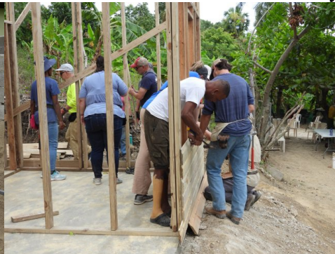
Applying siding boards
