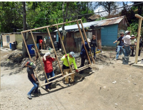
Front entrance wall arriving
