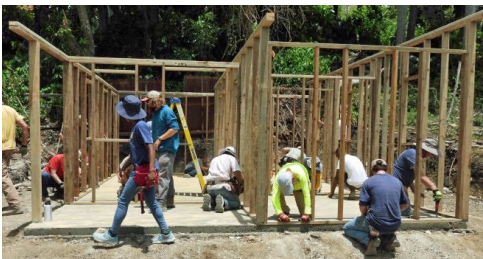
Nailing walls to concrete floor
