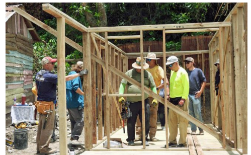
Inserting front entrance wall
