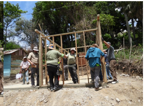
Front bedroom wall inserted
