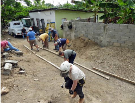
Getting 2x4 forms ready for other uses
