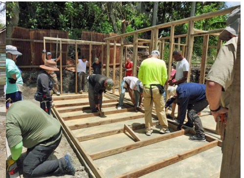
Splicing of south wall
