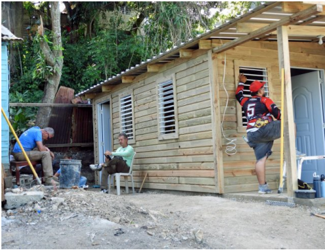
Corner and openings with trim boards
