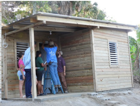
First nail in Casas plate by our team
