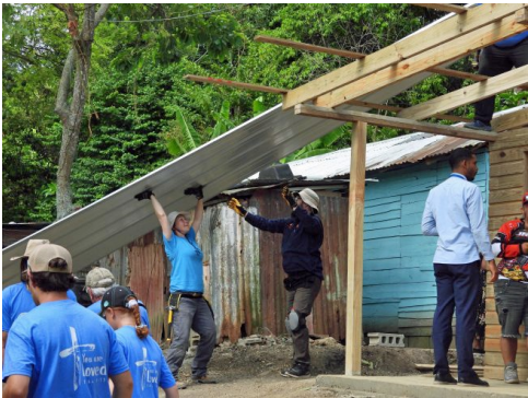
Metal roofing going up
