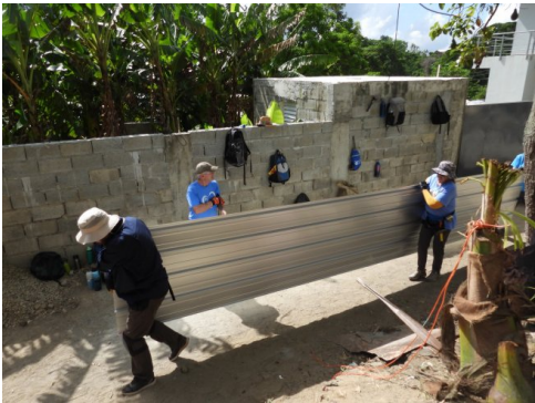
Then the roofing sheets came quickly
