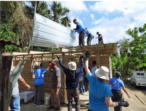
and were installed quickly
