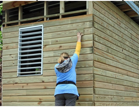
Hole-filling caulking is applied inside
