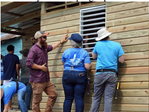
Installing the front window
