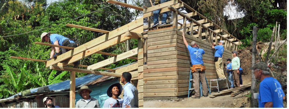
Attaching horizontal roof beams
