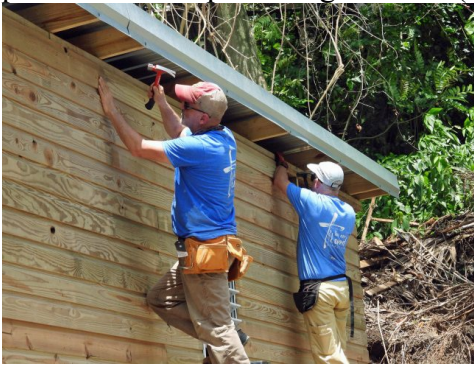
Finishing north siding
