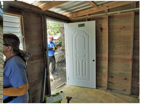
Installing rear door
