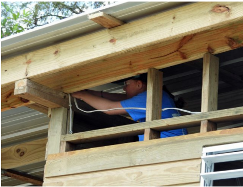
Adjusting more electrical wires
