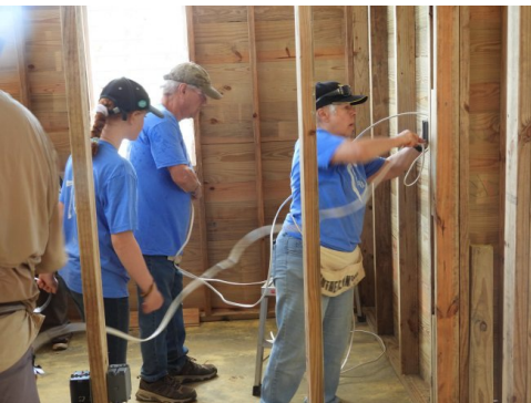
Installing electrical wires
