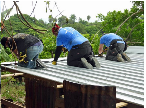
Installing the top roof edging
