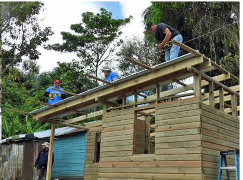
Screwing down the metal roof
