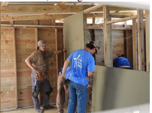
Installing fiberboard interior walls
